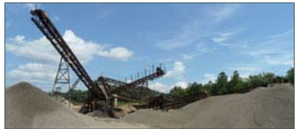
Sand & Gravel Plant
